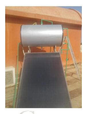
The water solar heaters covers all the guest rooms which reduce about 5000 kw/day (When using Electric Water Heaters)
